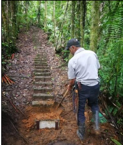
Luis Arana repairs steps on the Catarata (waterfall) trail at Pocosol.
